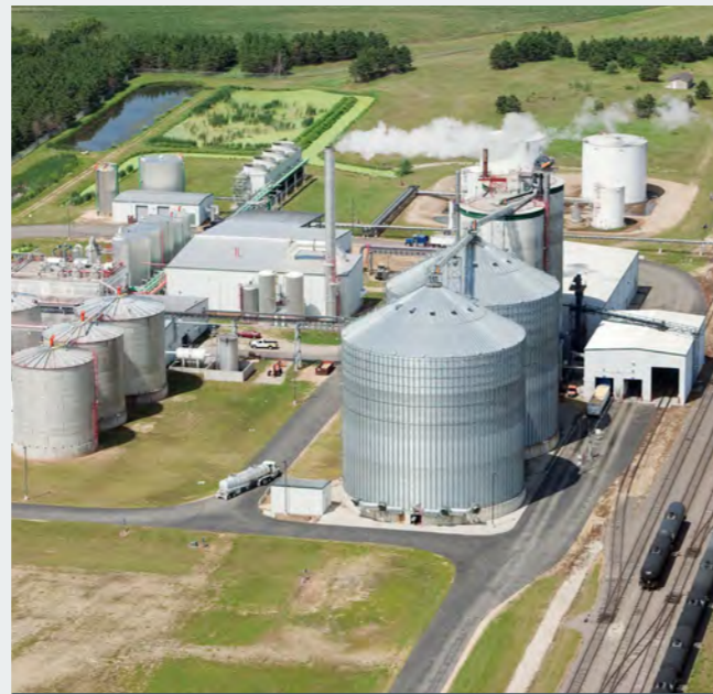
RENEWABLE ENERGY PLANT
