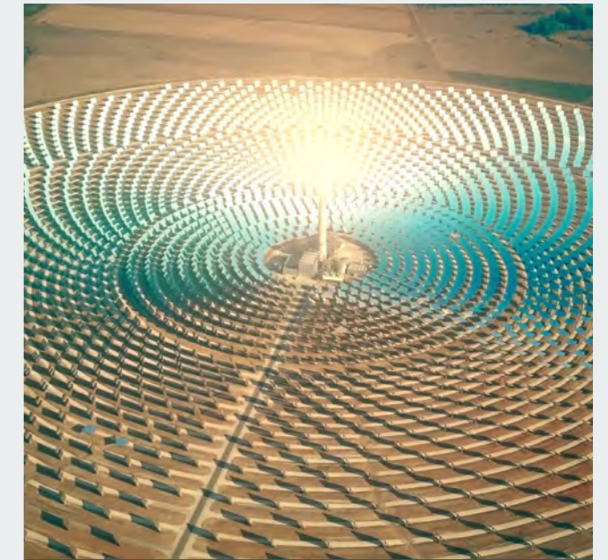
150MW CONCENTRATED SOLAR POWER PLANT
